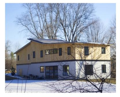
The home, designed by architect Christopher Smith, won an award from Efficiency Vermont for comprehensive efficiency in residential new construction. It combines insulation, air tightness, energy efficiency, and solar exposure. The cold-climate heat pump paired with the solar panels results in a house that is heated with renewable energy.
